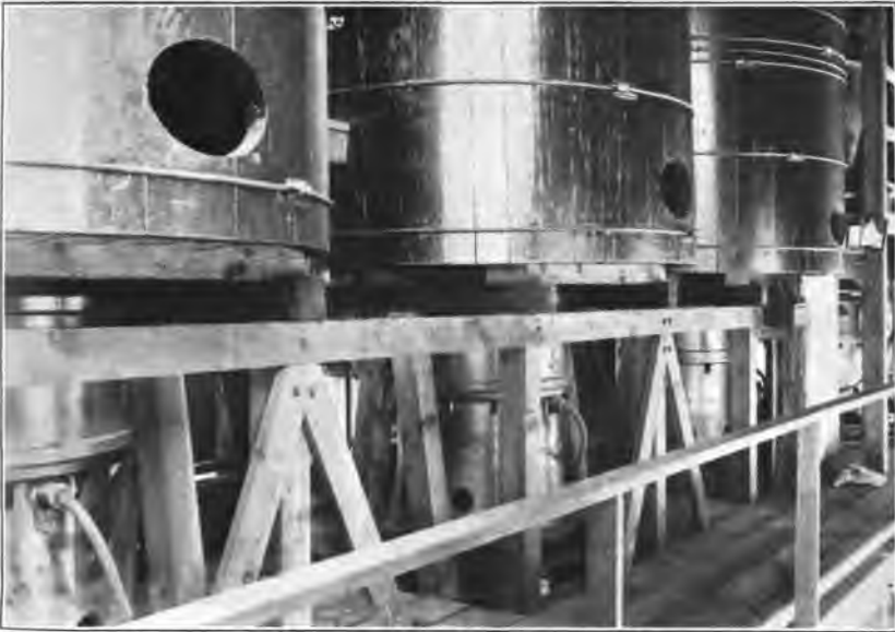
A. LOWER PART OF SETTLING TANKS, WITH EARTHENWARE FILTERS BELOW.
